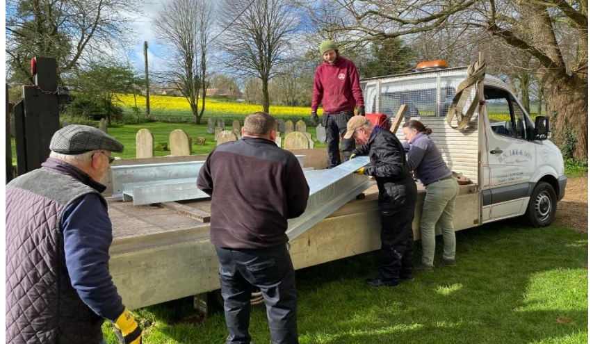
Unloading steel beam sections under the instruction of Bellhanger, Kit
