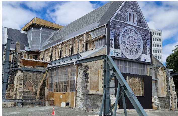
Christchurch Cathedral, awaiting reconstruction
