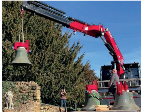
Bell 3 with canon-retaining headstock
