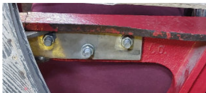
Frame showing over-plating repair
