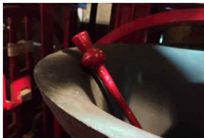
The new clapper in the tenor bell
